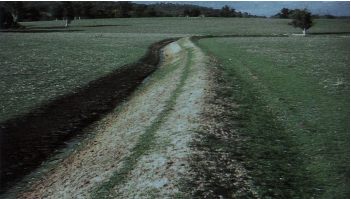
Figure 7.2 Reverse interceptor drain (from (McFarlane and Cox 1990))
