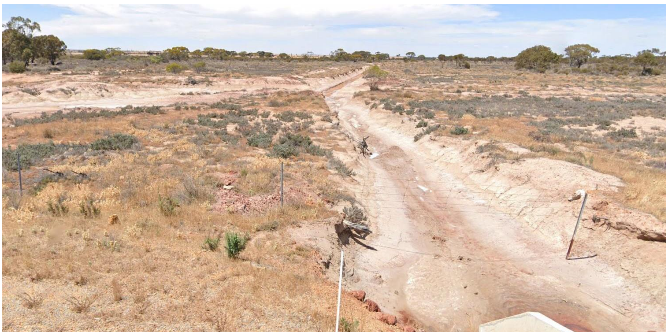
Figure 7.7 Typical groundwater drain in the Liebe Group salinity project catchment. From Google™ Streetview™
